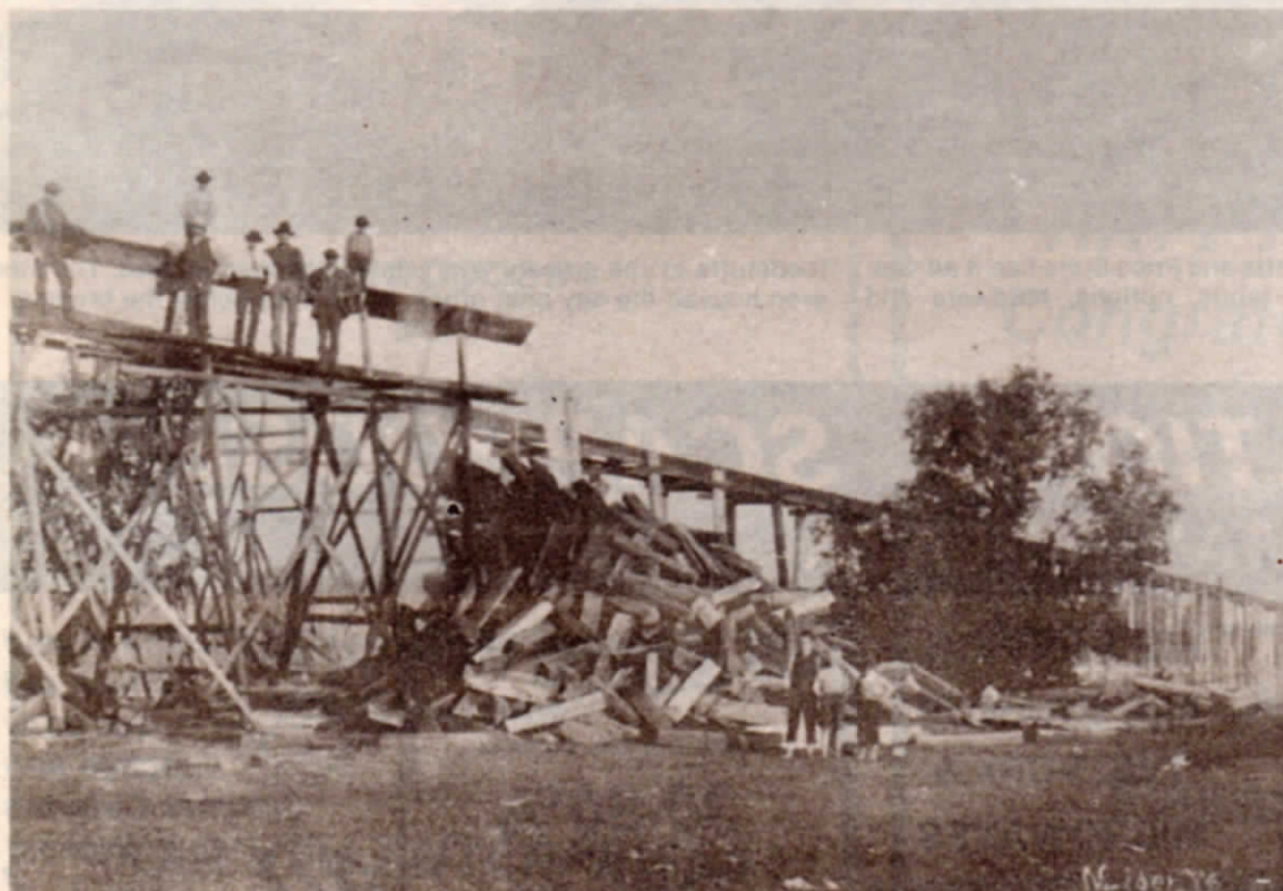
BRINGING DOWN LOGS —This flume brought logs down from the woods to the Wickstrom Planing Mill in Scappoose using water from Scappoose Creek. The mill was located close to the current location of the Scappoose Fire Station.
