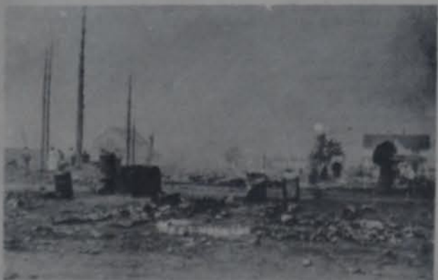
THESE TWO PICTURES show the destruction wrought by the 1915 fire which consumed the larger part of the city's commercial district from the Watts and Price Store South to where Crandalls
