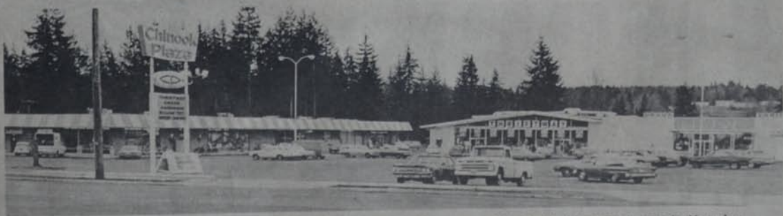
THE CHINOOK PLAZA is the latest completed shopping area in Scappoose. The latest tenant completed construction within the
