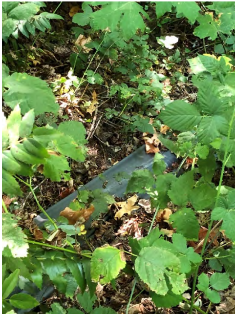
Site location: 16 Photo number: IMG_0680 Description: Storm sock at top of ravine
