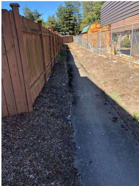
Site location: 8 Photo number: IMG_0710 Description: Overflow path behind home looking north/north west between homes.
