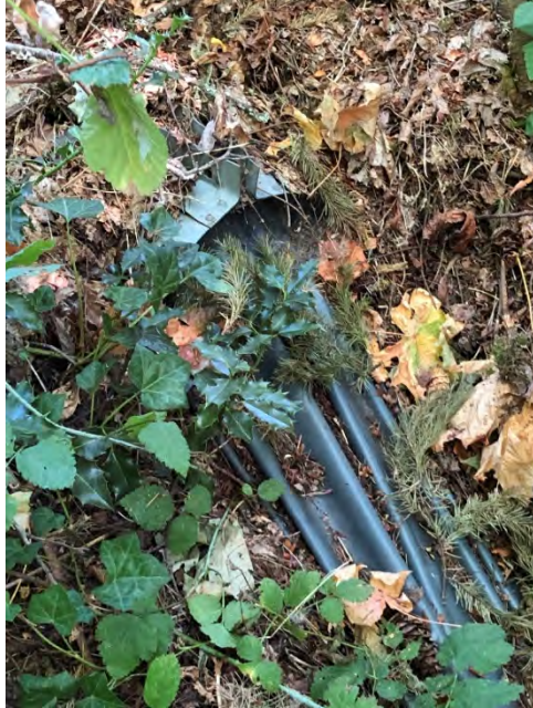
Site location: 16 Photo number: IMG_0681 Description: Storm sock at end of pipe
