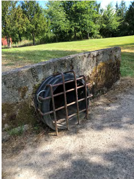
Model ID: PND03_N01 Photo number: IMG_7924 Description: Inlet structure into pipe through Miller Park.
