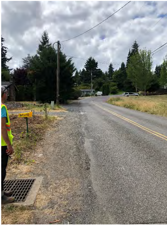
Model ID: SSC15_D03 Photo number: IMG_7907 Description: Area-drain and junction SSC15_D03, looking west up JP West Rd
