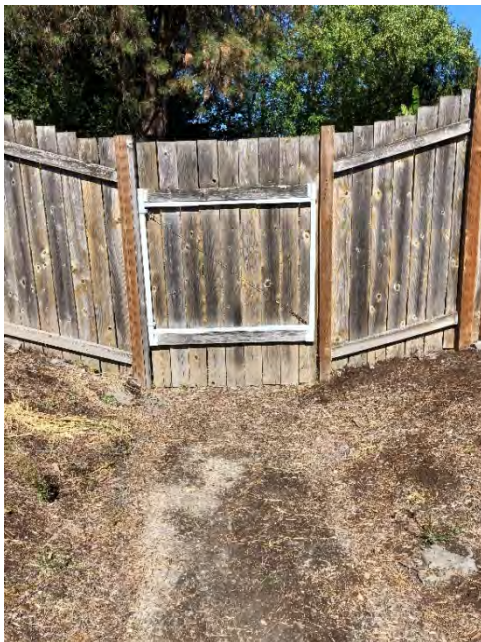
Site location: 8 Photo number: IMG_0708 Description: Overflow path behind home looking north.
