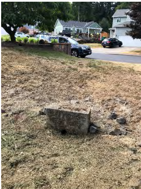
Facility Name Goss Subdivision Photo number: IMG_7914 Description: Inlet structure DS of WQ manhole into facility
