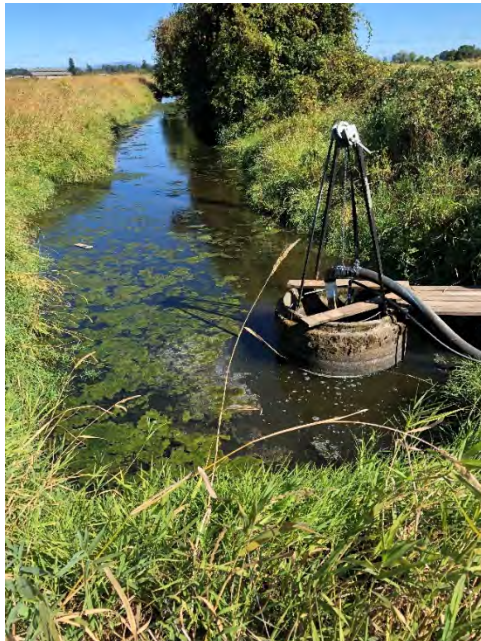
Site location: 30 Photo number: IMG_0722 Description: Outfall of ponds and SDIC drainage looking east.
