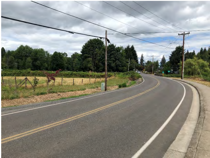
Model ID: SD0591 Photo number: IMG_7896 Description: Most downstream ditch to outfall, which is covered by overgrown bushes.
