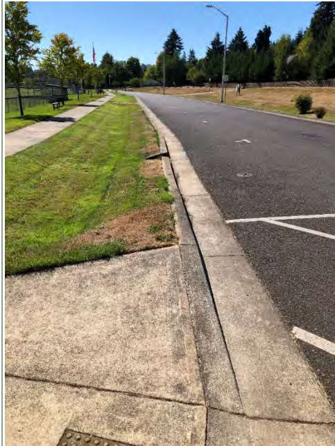
Site location: 20 Photo number: IMG_1798 Description: Veterans Park swale looking south.
