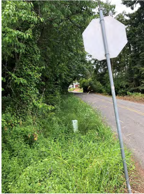
Model ID: SD0588 Photo number: IMG_7903 Description: Ditch on south side of Keys Road
