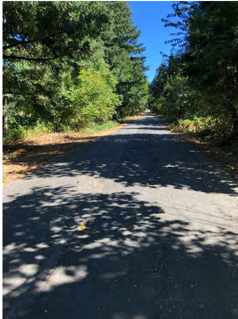
Site location: 13 Photo number: IMG_0699 Description: Existing path adjacent to large linear channel/ditch that is known to have high infiltration rates.
