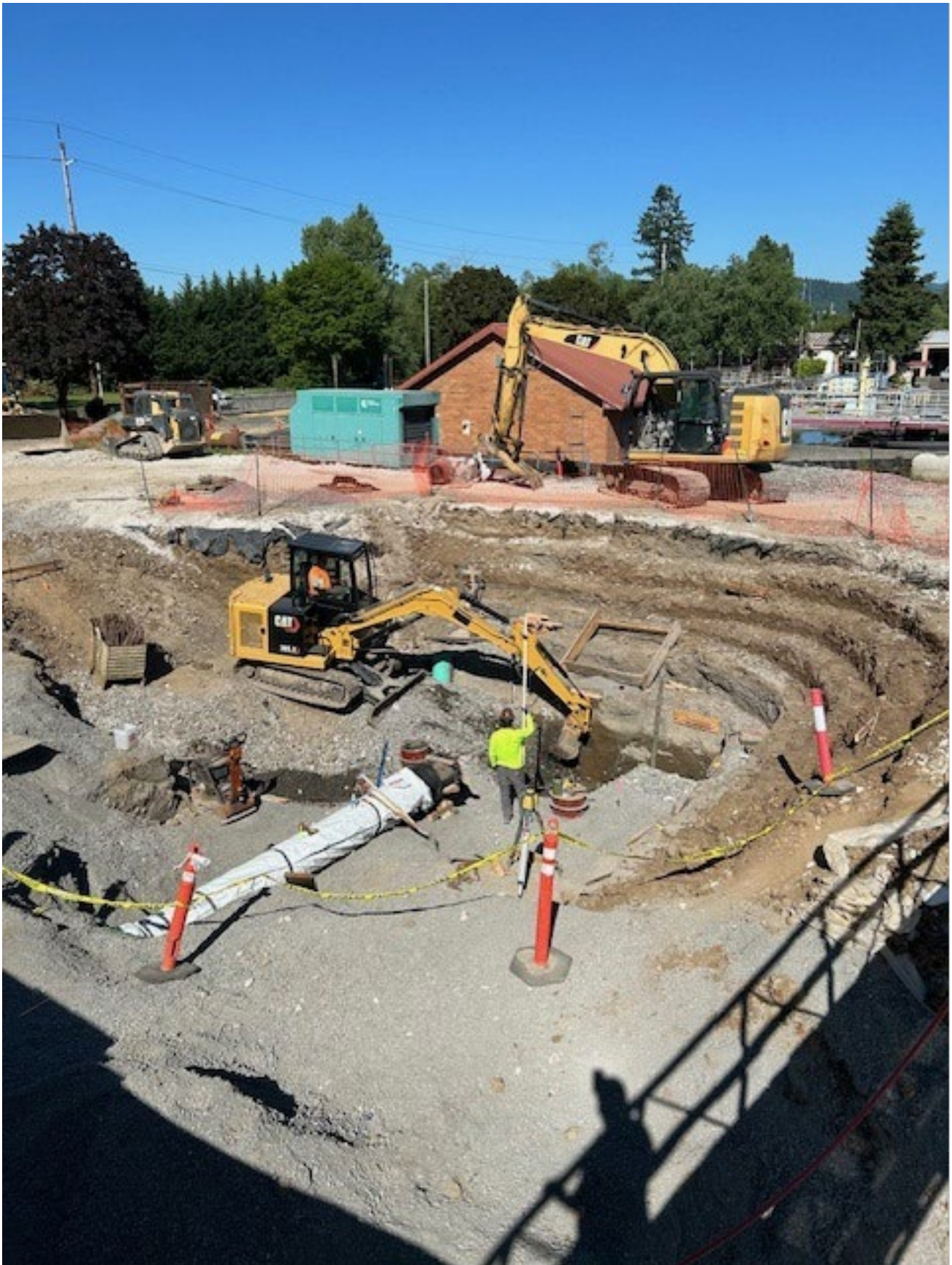
Figure 2 Wastewater Mixed Liquor piping
