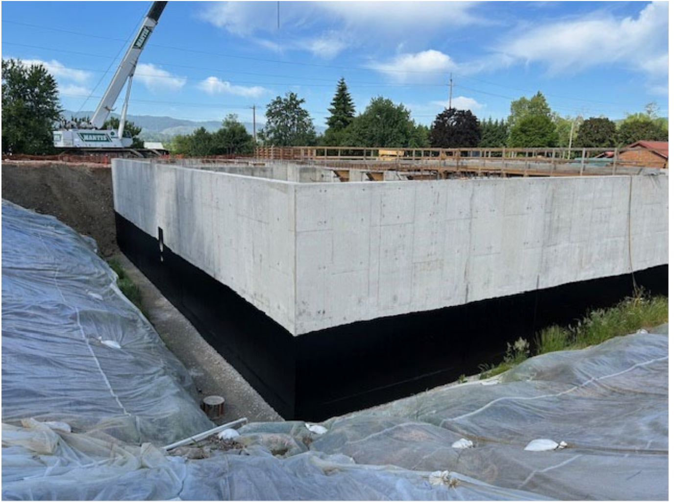
Figure 1 Wastewater Aeration Basin exterior coating
