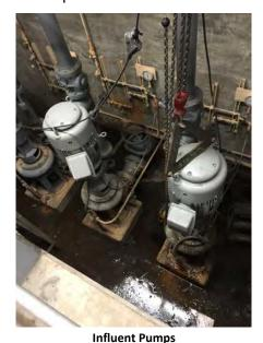
An overhead crane is located above the influent pumps for maintenance and removal. A sump pump, located in the southwest corner of the dry well, is used to remove water and pumps it to the wet well. It has been replaced twice in the past 10 years. There was also a large amount of moisture near the control panels. It is also likely that the number of air exchanges in the Headworks do not meet NFPA 820 requirements for an unclassified environment.
