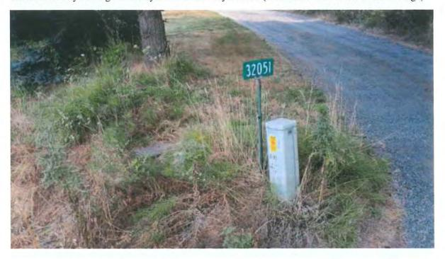
Meter vault too small for meter/reducing valve
