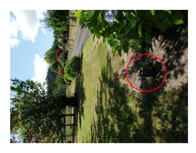
Cross connection; downspout on front porch smoking 8. 52895 NE 7<sup>th</sup> St
