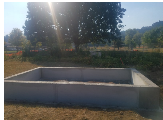
Restroom construction starting at Chief Concomly Park
