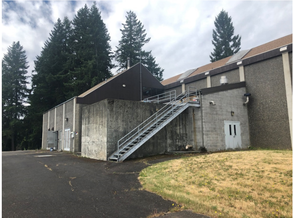
Photo 4: Filter 3 is the exposed masonry block room and cast-in-place tank Treatment Building addition at Keys Road.
