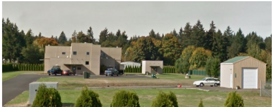
Photo 1: Overview of Miller Road WTP Buildings.
