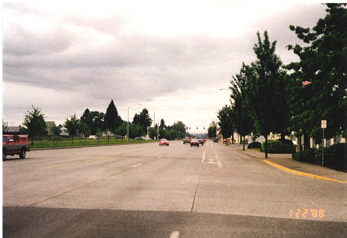
View of Highway 30 @ Watts Street looking south - Existing Conditions
