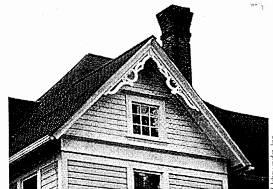
Scappoose historic building
