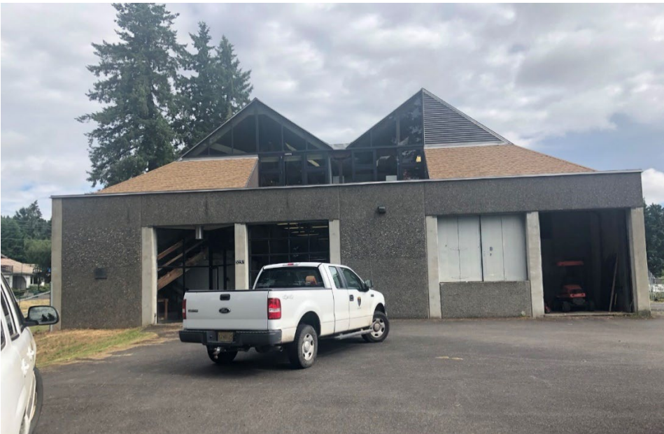
Photo 3: Keys Road Treatment Building main entrance complex configuration with large openings.
