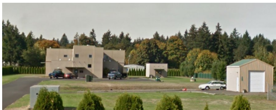
Photo 1: Overview of Miller Road WTP Buildings.
