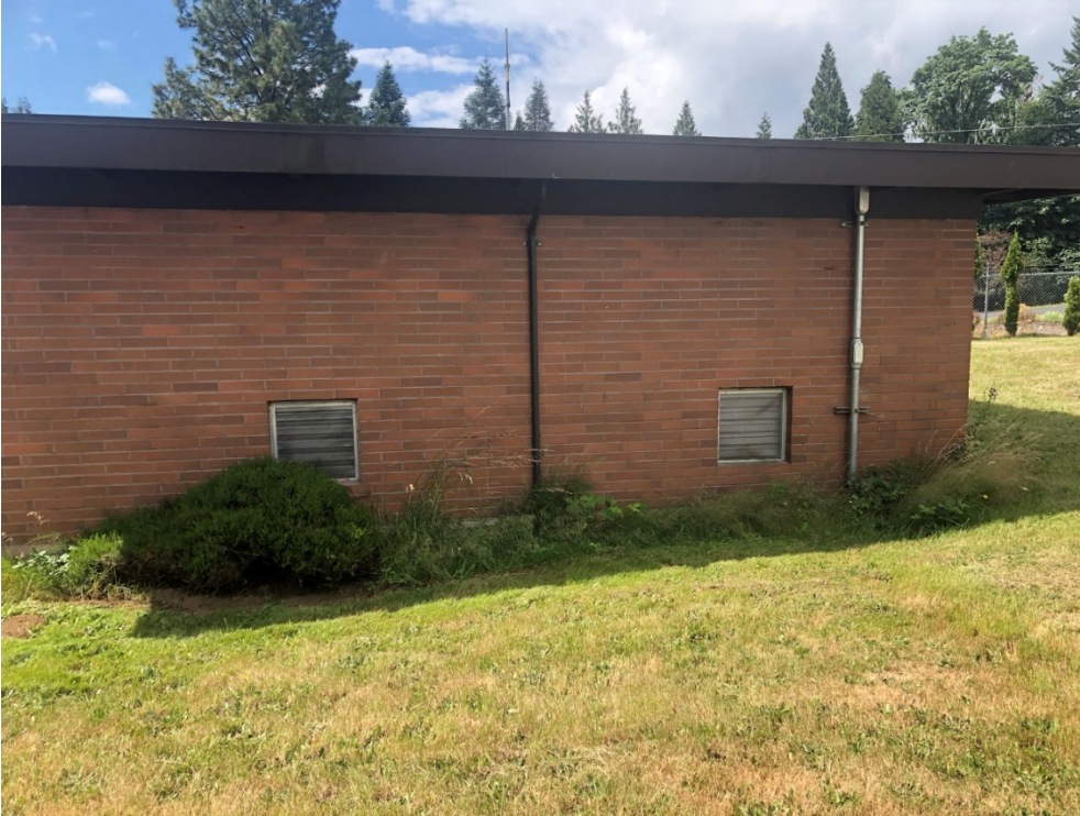
Photo 10: Keys Road Pump Station, record drawings were not available for review.
