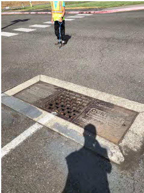
Model ID: N/A Photo number: IMG_7932 Description: CONTECH device in parking lot to south of HS Way.
