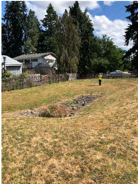
Facility Name Westview Subdivision Photo number: IMG_7928 Description: Looking south into facility at end of Erin Dr.
