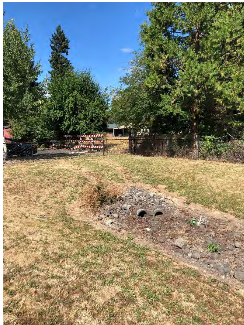
Facility Name Westview Subdivision Photo number: IMG_7929 Description: Looking northeast, facility outlet shown.
