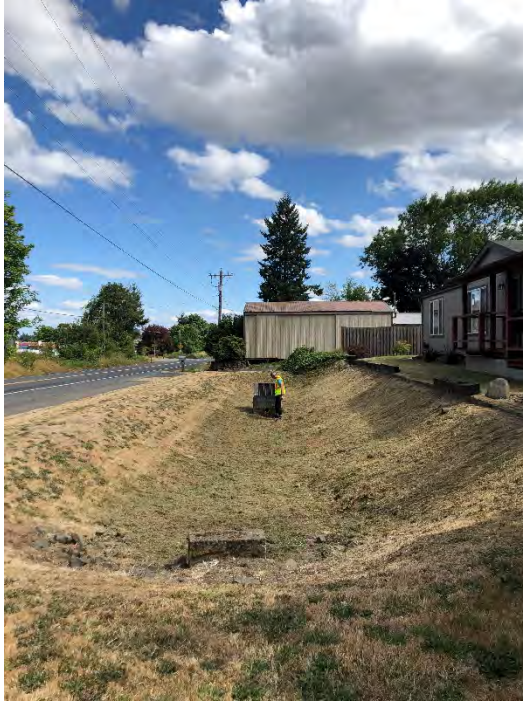
Facility Name Goss Subdivision Photo number: IMG_7913 Description: Full length of facility, looking north from Manor
