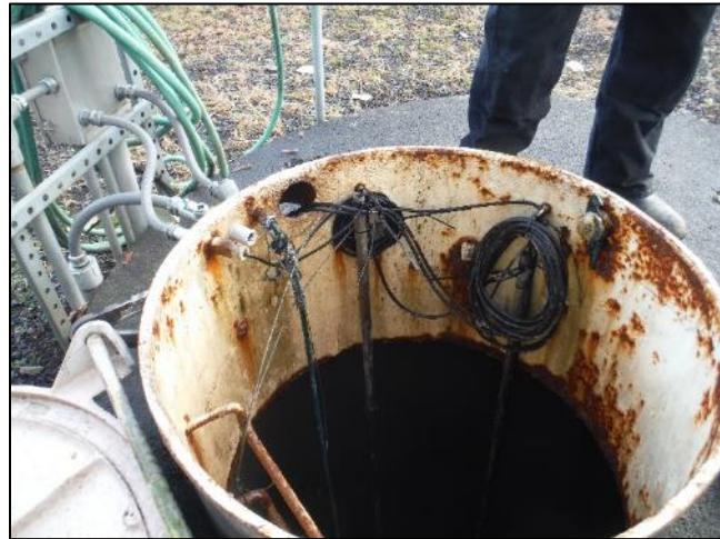
Smith Road Pump Station
