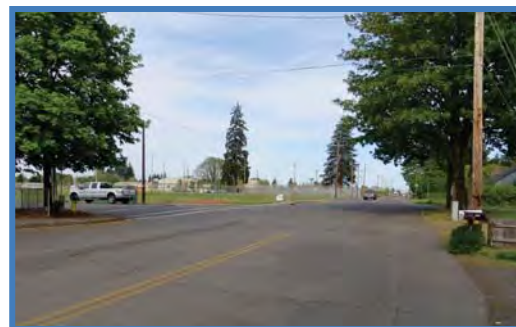
Gaps in Sidewalks on Collector Roadway
