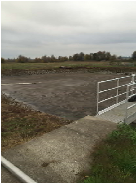
Biosolids Storage Lagoons
