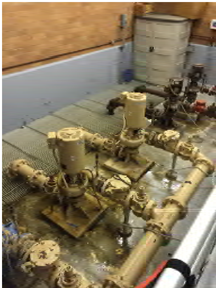
Sludge Pumping Building
