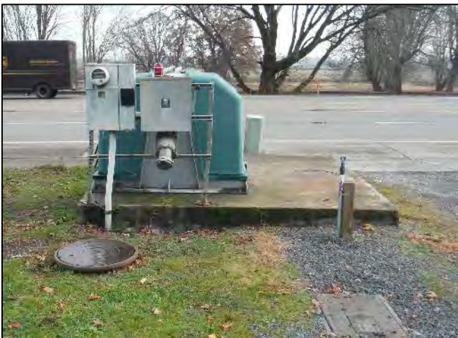
Highway 30 Pump Station
