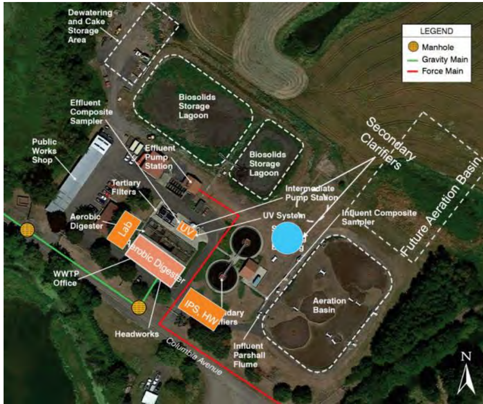
Figure 1. Scappoose WWTP Aerial Photo.
