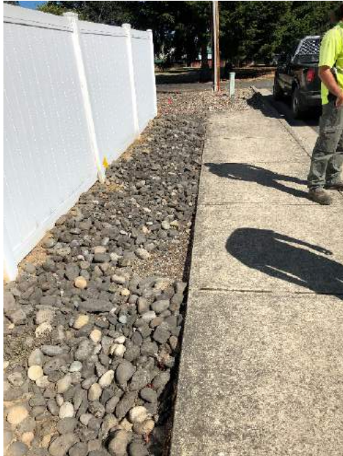
Site Location: 3 Photo number: IMG_0718 Description: French drain looking east along Elm Street.
