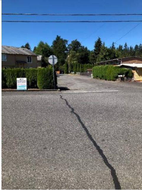
Site location: 2 Photo number: IMG_1802 Description: Area drain looking west.
