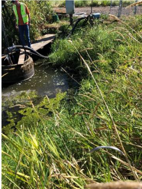
Site location: 30 Photo number: IMG_0721 Description: Outfall of pond system into SDIC drainage system
