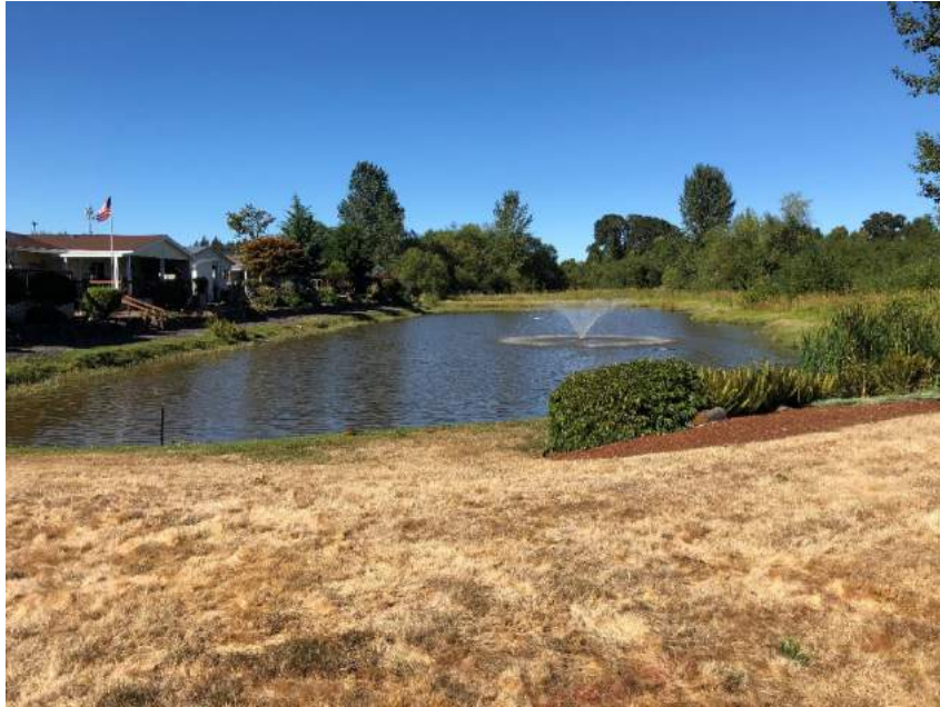
Site location: 30 Photo number: IMG_0725 Description: North pond looking north. Trail along pond floods during large events.
