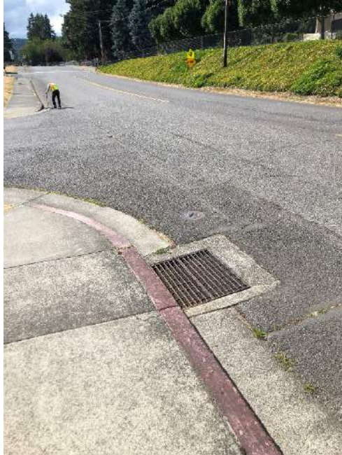
Model ID: DW37_CB02 Photo number: IMG_7933 Description: Catch basin in curb at corner of parking lot, looking west. Pipes visible in basin from east, west, and south.
