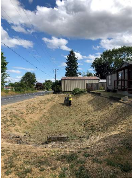
Facility Name Goss Subdivision Photo number: IMG_7913 Description: Full length of facility, looking north from Manor
