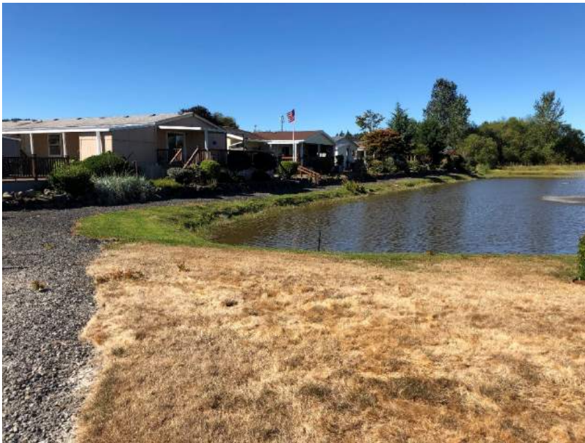
Site location: 30 Photo number: IMG_0728 Description: North pond looking north. Trail along pond floods during large events.
