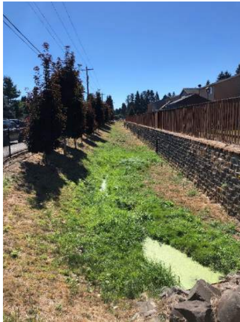
Site location: 28 Photo number: IMG_0686 Description: Large private infiltration facility that receives runoff from multiple neighborhoods and private property as well as roads and public spaces. Looking south.
