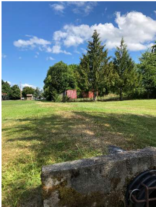
Model ID: SD0724 Photo number: IMG_7926 Description: Mound conveying pipe through Miller Park.
