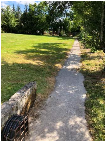
Model ID: PND03_N02_PND03_N01 Photo number: IMG_7925 Description: Drainage pathway that conveys upwelling from CB at sunset loop through to Miller Park. Inlet structure into pipe through Miller Park.
