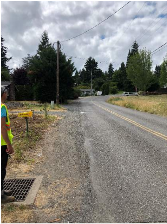
Model ID: SSC15_D03 Photo number: IMG_7907 Description: Area-drain and junction SSC15_D03, looking west up JP West Rd
