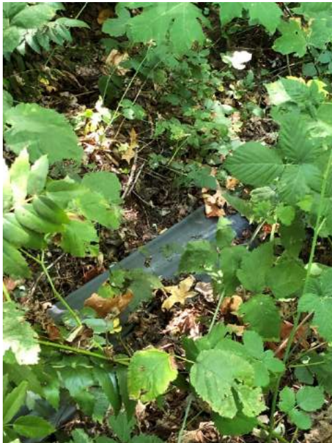
Site location: 16 Photo number: IMG_0680 Description: Storm sock at top of ravine
